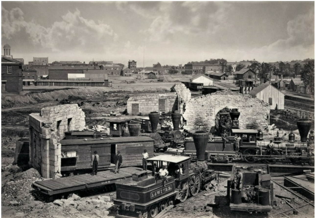
Atlanta, Georgia after the end of the American Civil War, railroad roundhouse in ruins – George N. Barnard, U.S. Library of Congress, Wikimedia
